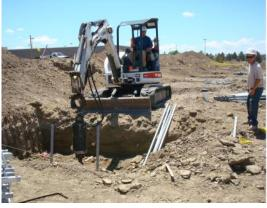
The ECP Model TAF-175 Torque Anchor<sup>176</sup> solid square shaft helical pile was installed at each placement to a required minimum depth of 45 feet below grade. The pile configurations varied due to soil borings encountering very dense soils at 10 to 15 feet deep on a portion of the site.
