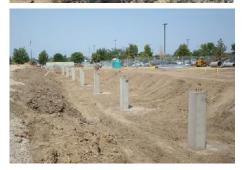
At these placement locations, a smaller plate configuration was used to allow the pile to reach the target depth before experiencing excessive shaft torsion. The installation shaft torsion 8,700 foot-pounds was needed to provide a service load of 43,500 pounds with a factor of safety of 2.0.
